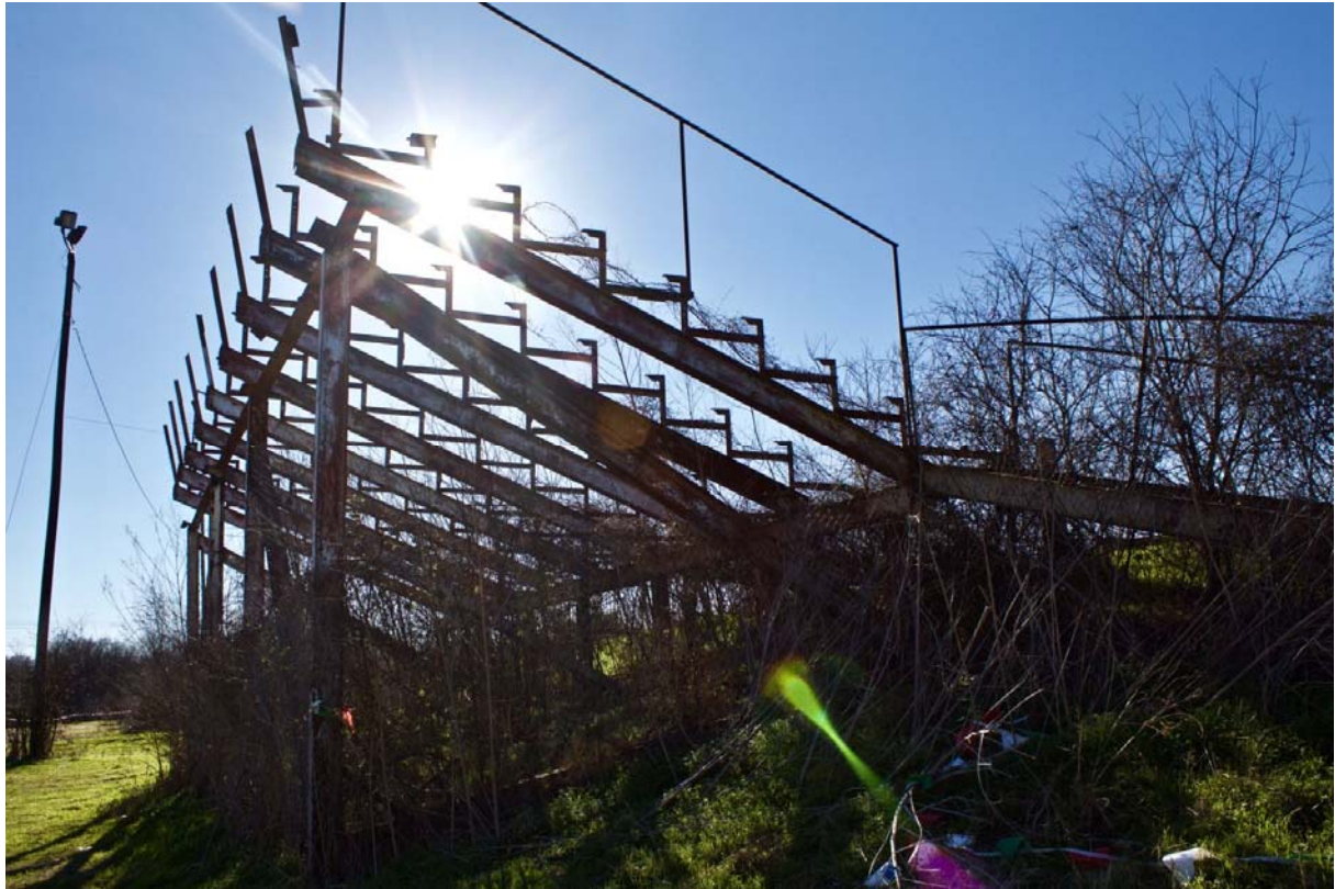
The backstretch grandstands, with a ramp now completely twisted with rust and age.
